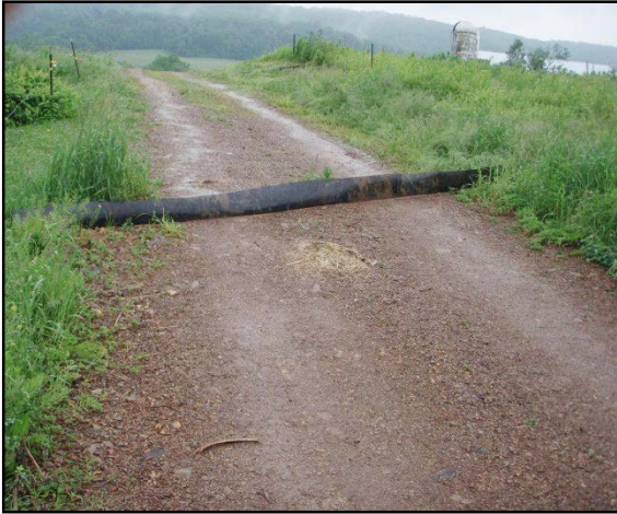
Completed Conveyor Belt Diversion
