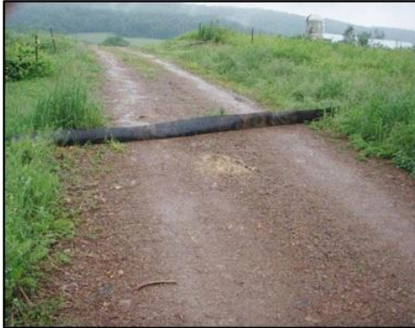
Completed Conveyor Belt Diversion
